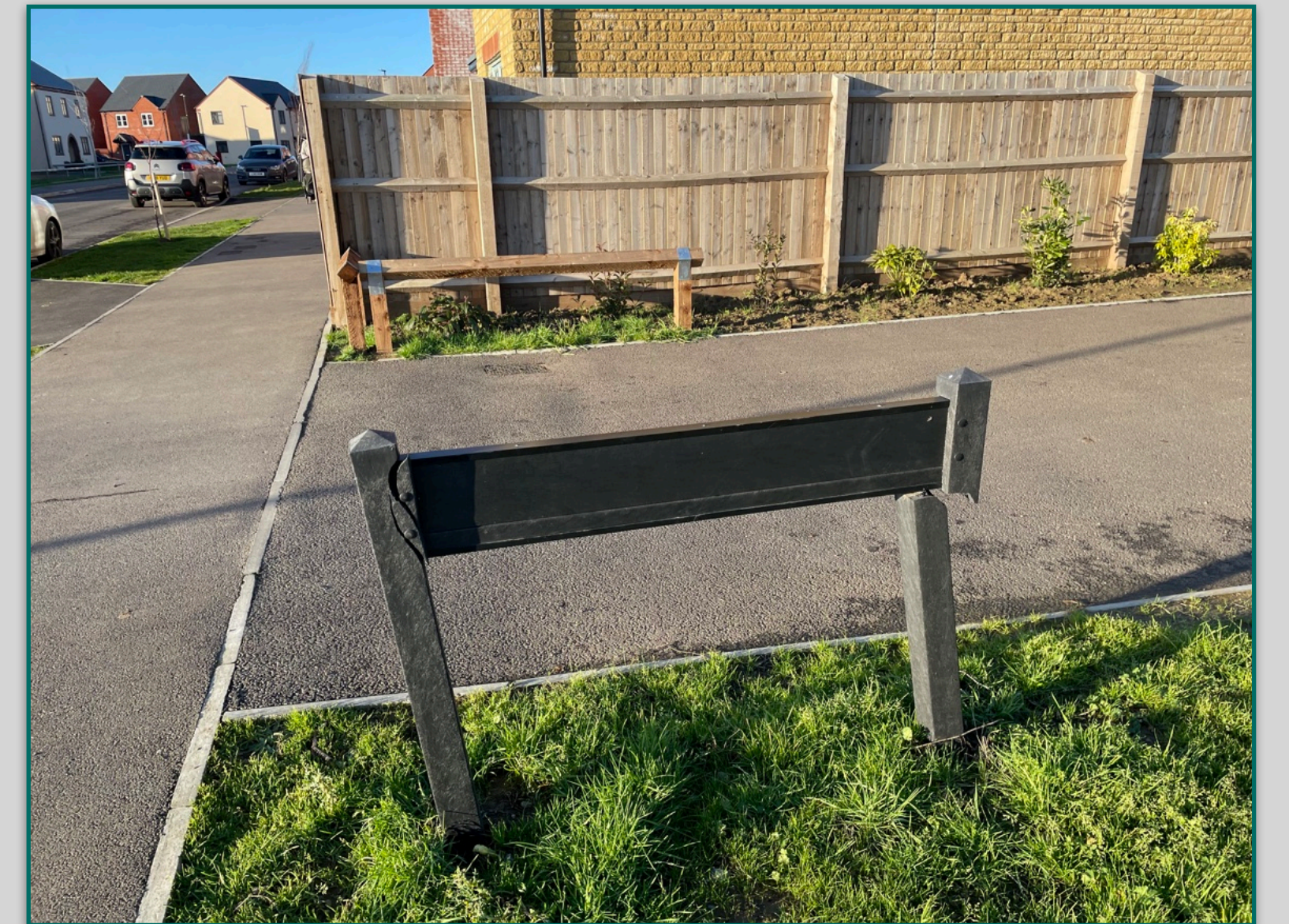
Broken Street Sign
